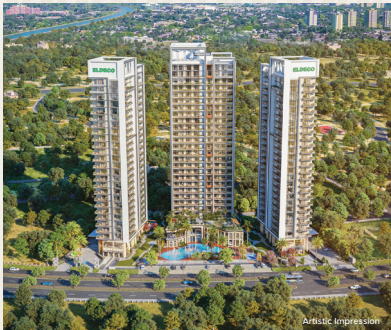
Eldeco Trinity, Gomti Nagar Extension, Lucknow
